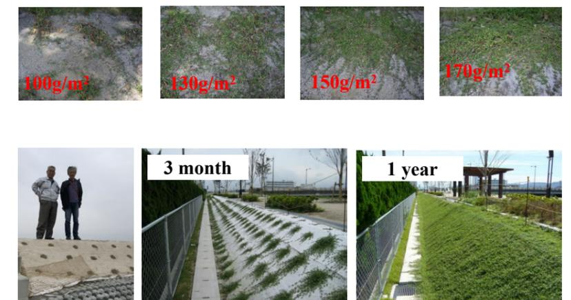
Figure 4. HydroCycle culture in dryness embankments. Upper panels: Cotton sheet thickness effect on plant growth. Lower panels: slope greening construction (greencosmo construction) method mulching with cotton sheet (SoilCott Registered Trademark).
